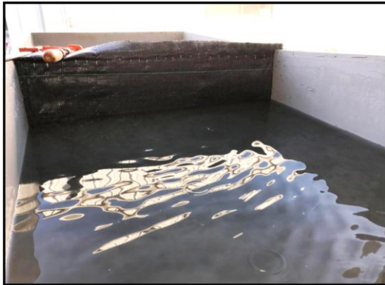
Typical Upstream View - With Sediment-Laden Discharge
