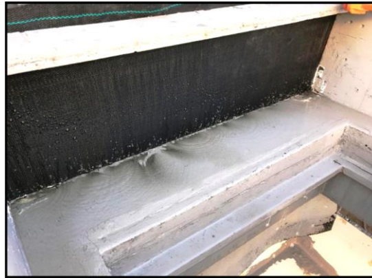
Typical Downstream View - With Sediment-Laden Discharge
